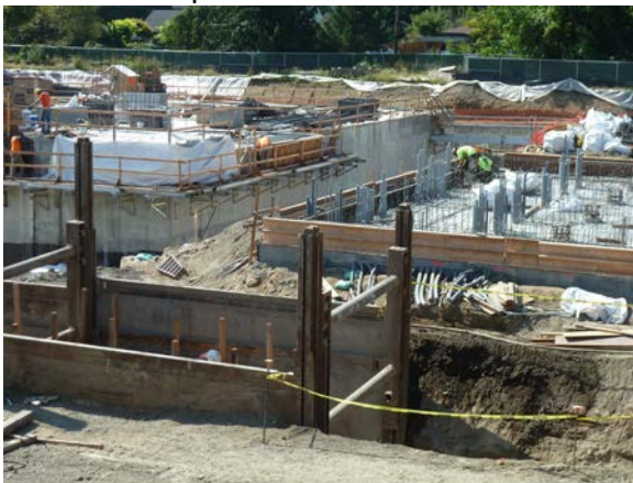
Foreground: Excavated trench and shoring in place for the 48" overflow pipe at the WTP. Electrical building foundation and clearwell in the background.
