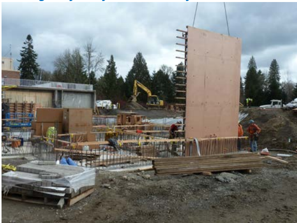
Forming the first of the ballasted floc. walls this week
