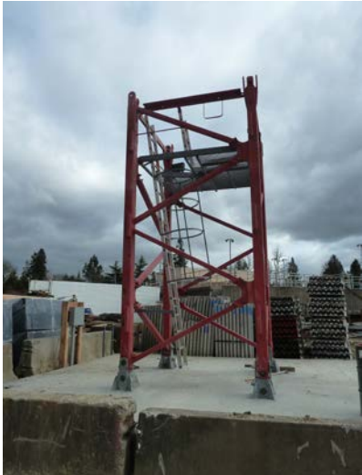
Preparing the tower crane foundation
