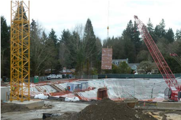
Forming walls in the clearwell on 2/25/14
