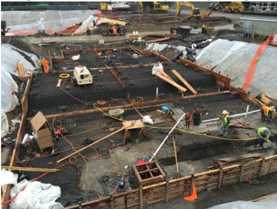
Preparing the ballasted floc. base prior to pouring concrete
