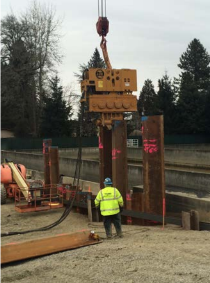
Installing sheet piles to support the solids storage tank
