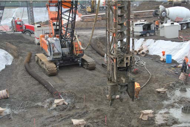
Drilling auger cast piles in the ballasted flocc. area (below)
