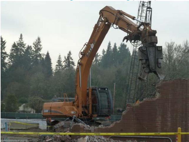
Demolishing the lime building (below)
